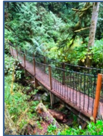
Failing Whiskey Creek Bridge Built on old hemlock log.
