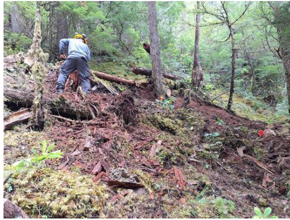
Getting rid of a thick layer of "duff" (organic material)
