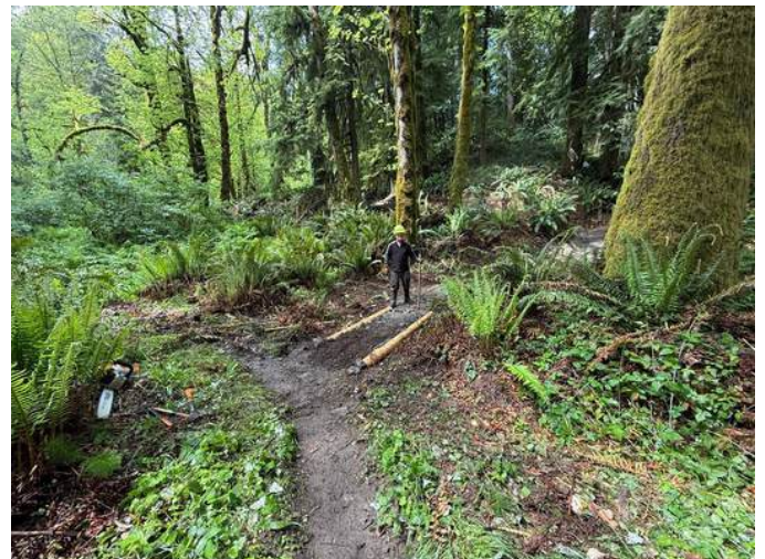
Going down around the climbing turn towards the bottom entrance. You can see material that was poured on top of the clay. Also, the climbing turn itself was constructed by tossing a huge pile of logs and small trees to give the turn a backdrop and soil supporter. Otherwise what we had was a huge, deep hole. (you can see it better in the lower left picture of the previous page).
