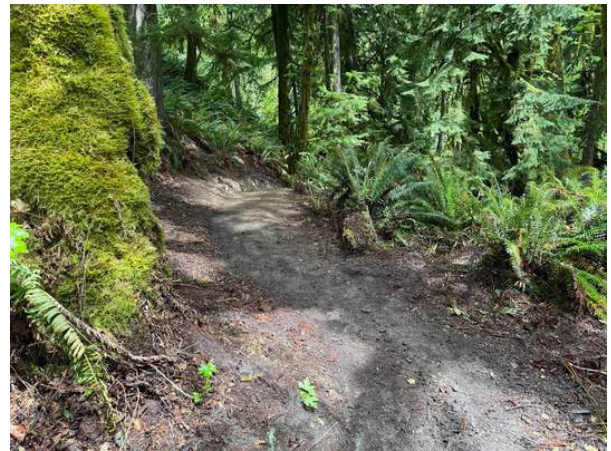
Part way down the trail. It's hard to tell here, but dozens of ferns were replanted and organic material tossed on the downhill edge, to give the trail a less recently-built look.
