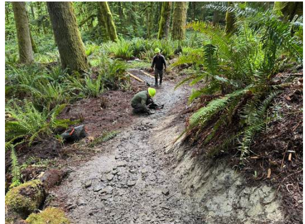
Going down around the climbing turn towards the bottom entrance. You can see material that was poured on top of the clay. Also, the climbing turn itself was constructed by tossing a huge pile of logs and small trees to give the turn a backdrop and soil supporter. Otherwise what we had was a huge, deep hole. (you can see it better in the lower left picture of the previous page).
