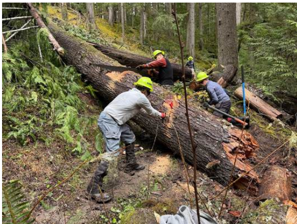
Working on two cuts at once, something you can do with crosscut saws because the cuts take a while on a tree of this size.
