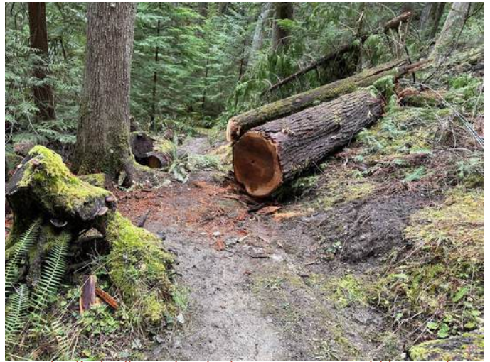
Finished! Ideally, and with chainsaws, we would have taken off a few more chunks on the foreground tree. The reason we left it like that is it is passable, and if we took off another chunk, the whole thing would have rolled into the trail. Sometime we will get rid of the rest of it, but today it was hugely better and we had miles to cover.
