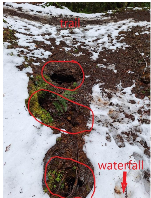
Water running under the trail around wood box culvert. Creating sinkholes.
