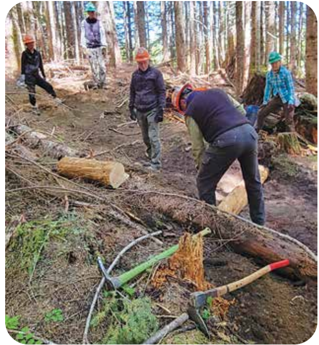
Washington Trails Association crew working on check steps on the Cinnamon Trail.
