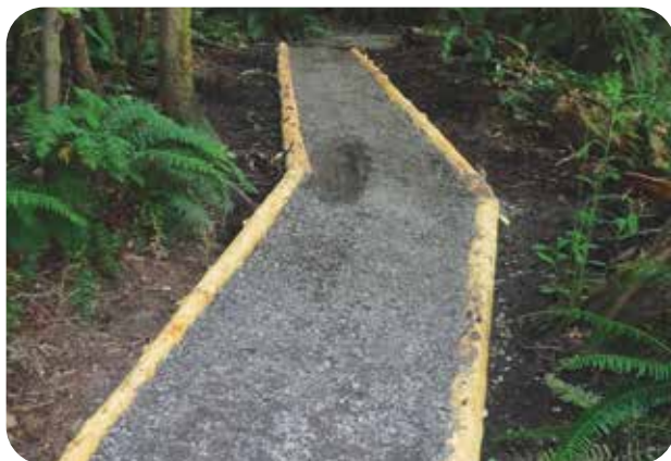
New area of completed turnpike.
