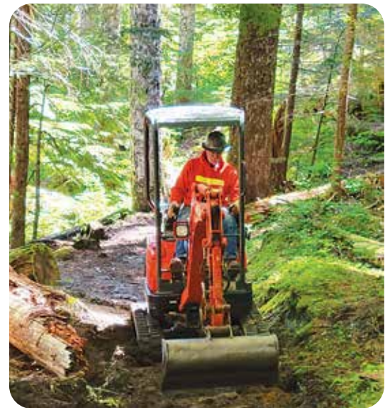
Tom Connors operating the excavator on the Cinnamon Trail.
