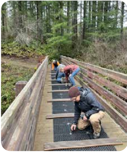
Setting mats on bridge.
