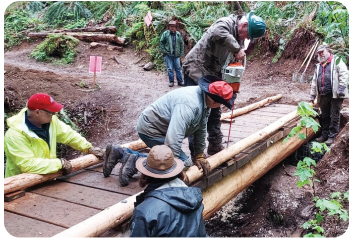
Attaching bull rail: Tom Mix using drill; Jim Hollatz holding rail in position. Other workers' names unknown.
