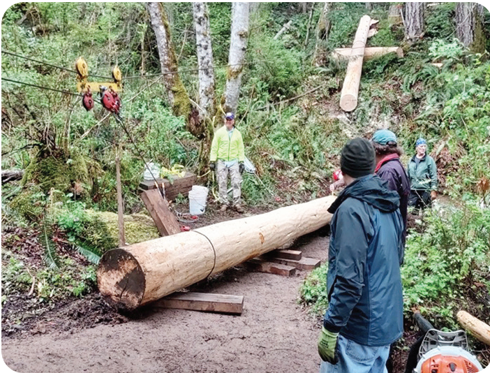
Using cables, pulleys, and Gripjoists, the stringer pieces are moved toward the bridge site using BCHW expertise.
