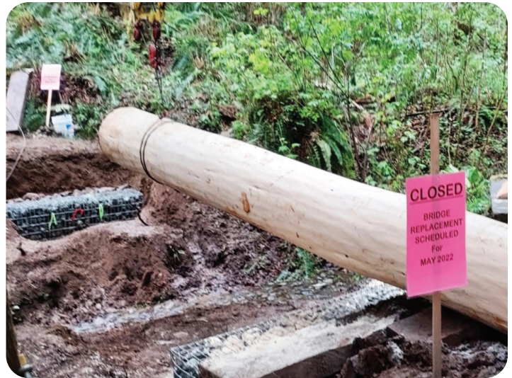
Using cables, pulleys, and Gripjoists, the stringer pieces are moved into place onto rock-filled gabion-basket foundation.
