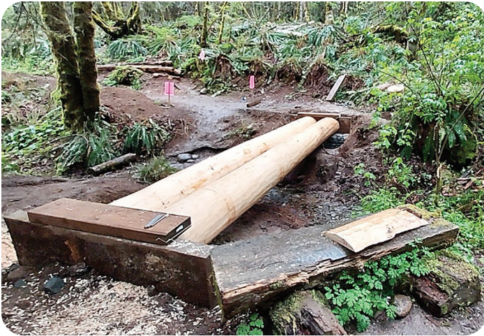
Stringers for the new bridge are in place and ready for decking.
