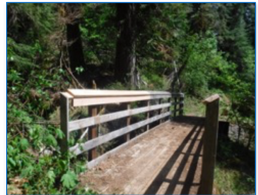
Bridge with repaired railings.
