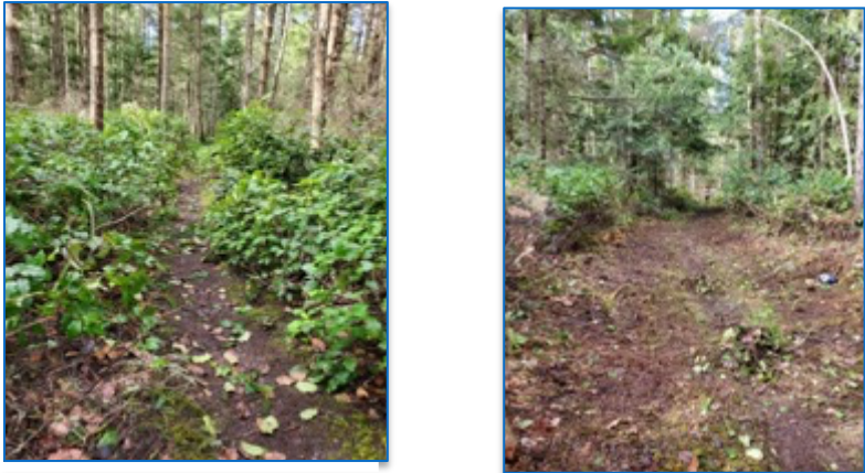
Before and After WCC Crew Trail Clearing
