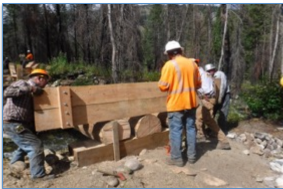
Installation of abutment.
