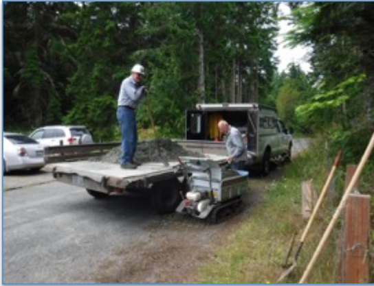
Loading gravel into the motorized totter.
