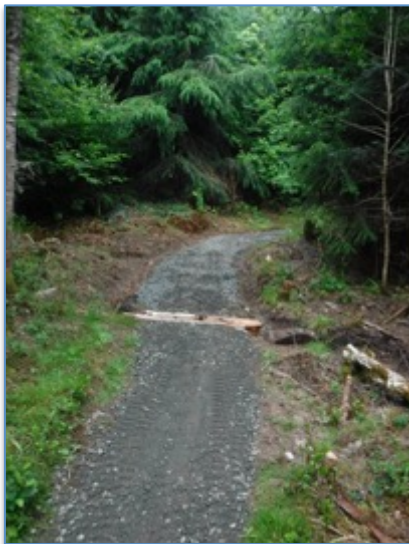
New drainage and gravel added to trail section.
