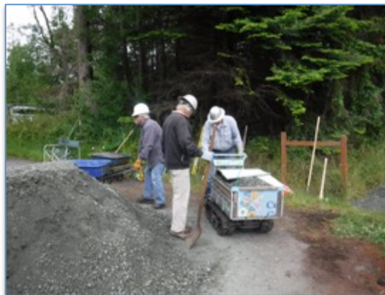
Power totter and wheelbarrows were used to move gravel along the trail.
