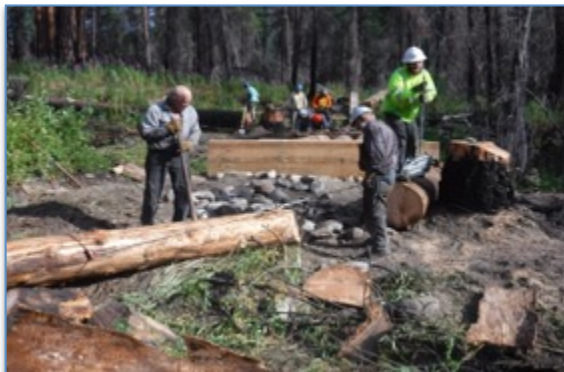
Logs used to build approach.
