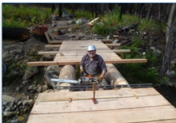
Installation of planking.
