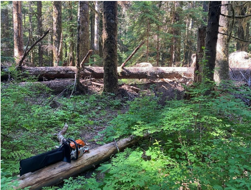
THIS IS THE LAST PROJECT WE SAW LAST SUMMER, WE HAD TO LEAVE THIS UNTOUCHED DUE TO NEEDING THE REMAINDER OF OUR SAW GAS FOR A LARGE PROJECT THAT FELL DOWN BEHIND US AS WE CLEARED UP THE TRAIL (WE HEARD ABOUT THAT FROM HIKERS). REBECCA WAS EAGER TO GET BACK TO THIS MESS THIS YEAR. THIS IS RIGHT BEFORE THE FORD ACROSS THE ELWHA. LOOKING SOUTH.
