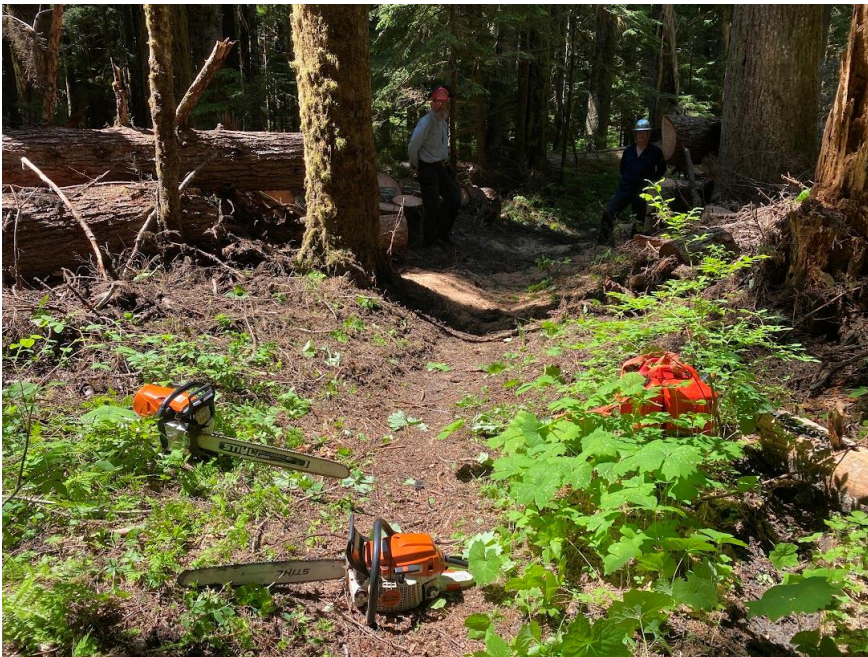
CLEARED! LOOKING SOUTH.
