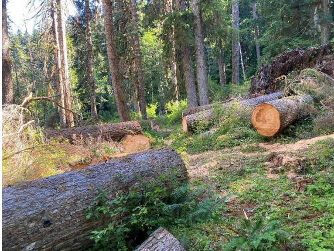
LOOKING NORTH BACK AT THE CLEARED PROJECT.
