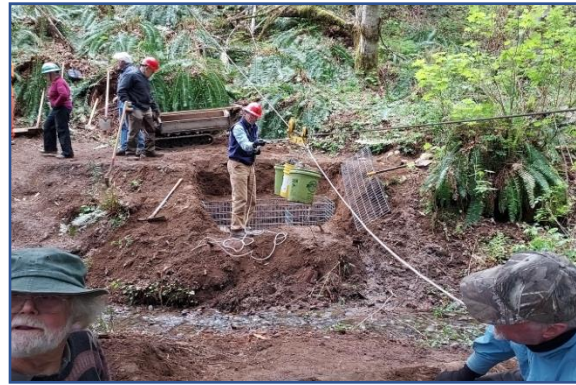
Moving rock to fill gabion baskets.
