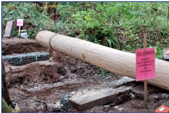
Placing the stringers on the gabion base.
