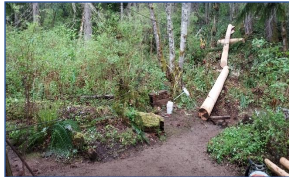
Sliding the stringer log pieces toward the bridge.
