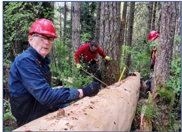
Peeling bark from the log that will become the new bridge stringers.
