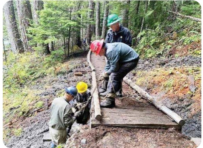
Shoveling in the muck, sawing old planks, clearing out the uphill ditch, using jacks to push up the puncheon and hold it in place – there were a lot of different jobs happening all at once. Rocks had to be collected. Off-site drainage work needed to be done.
