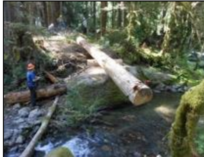
Rigging was used to move the log across the stream.
