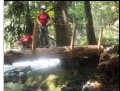
Installation of the hand rail along the log.
