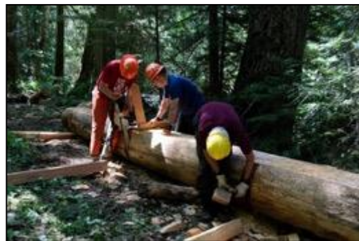
Slots being measured & cut for handrail placement.
