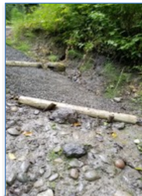
After the gravel was hauled, it was raked level to create a great approach to the creek ford.
