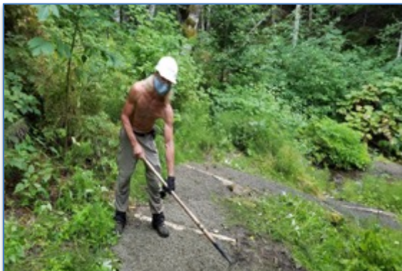
After the gravel was hauled, it was raked level to create a great approach to the creek ford.
