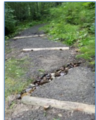
After the gravel was hauled, it was raked level to create a great approach to the creek ford.
