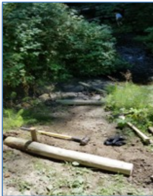
Curb logs installed by Buckhorn Range.
