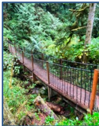
Failing Whiskey Creek Bridge Built on old hemlock log.
