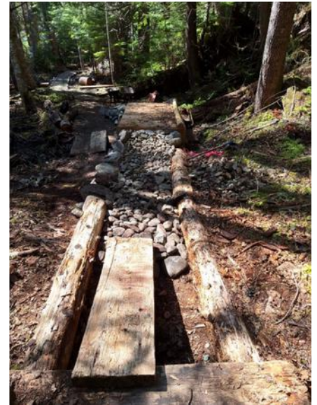
Work underway (end of next puncheon at bottom)
