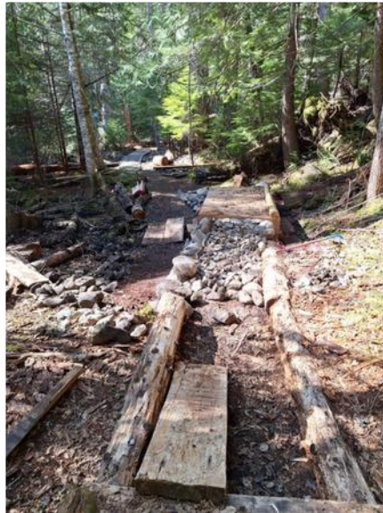
Work underway (end of next puncheon at bottom)
