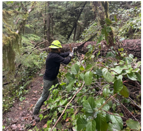
This one wasn't large, but it was fully suspended down below to the left off the trail. It started cracking and popping almost right away because of the weight of the tree down below. Once released, the piece to the left sprang up and AWAY from the sawyer (predicted, that's why I'm cutting from where I am and angling it to let the piece go in that direction) and then slid way down off the trail in a split second.
