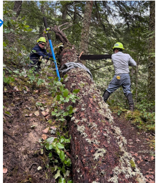
This tree had severe bottom bind due to the weight of that suspended rootball. It was also suspended down below to the right after it went off the trail.
