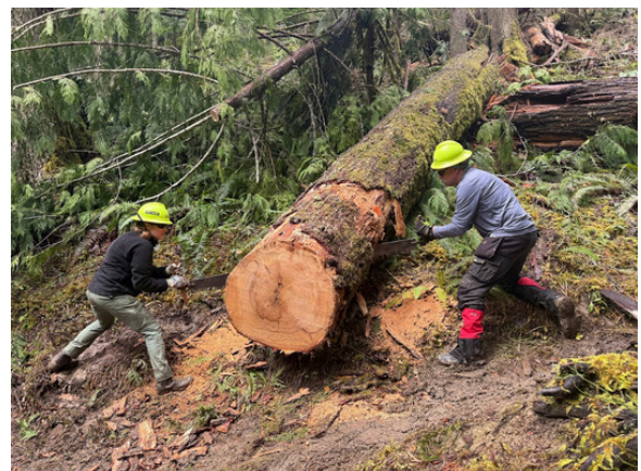
We really didn't have any unexpected difficulties to this project, other than the hillside (and the trail) in this area is wet clay. Extremely slippery. This made safe footing a challenge.
