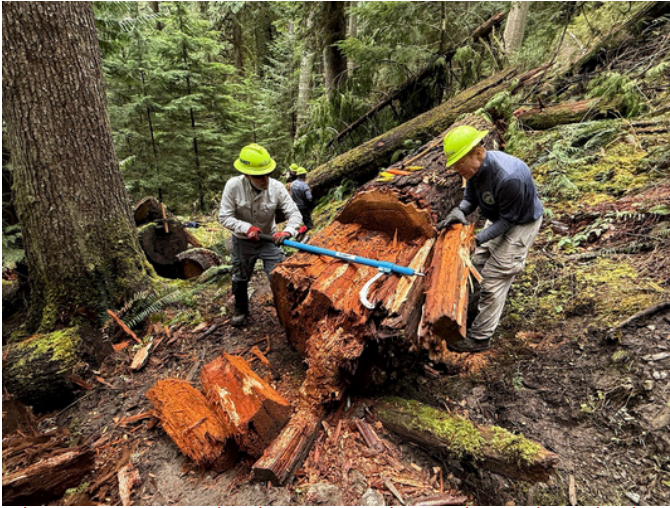
This one was completely rotten and waterlogged. We had to do a combination of sawing and breaking it apart.
