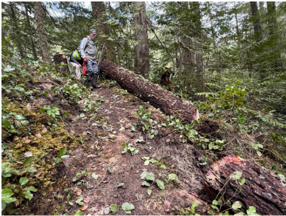
This one wasn't large, but it was fully suspended down below to the left off the trail. It started cracking and popping almost right away because of the weight of the tree down below. Once released, the piece to the left sprang up and AWAY from the sawyer (predicted, that's why I'm cutting from where I am and angling it to let the piece go in that direction) and then slid way down off the trail in a split second.
