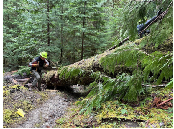
Getting started by single bucking with the smaller of the saws that we brought. (the guys with the bigger saw were finishing up an earlier project)
