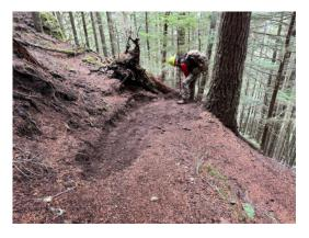
Left: this switchback was getting damaged by water seeping off the hillside. The water needed to be corralled and directed.
