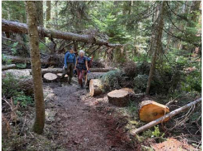
Later in the crew Eric did some skilled tread work. Barbara and Sonya pose on the new trail going around the rootball.
