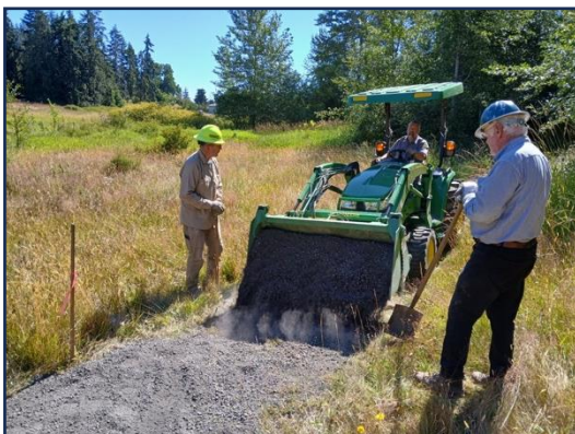
Hardening section of previous trail by adding gravel.
