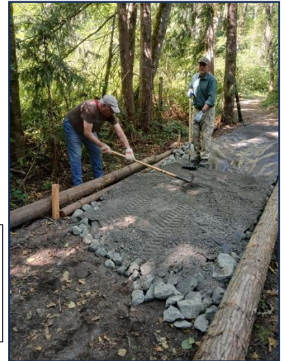
Spreading gravel layer.
