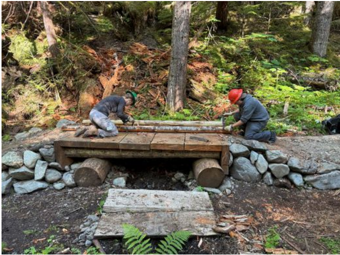
Prep bull rails (with upstream puncheon as worktable)
