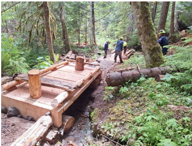
ready for ramps
