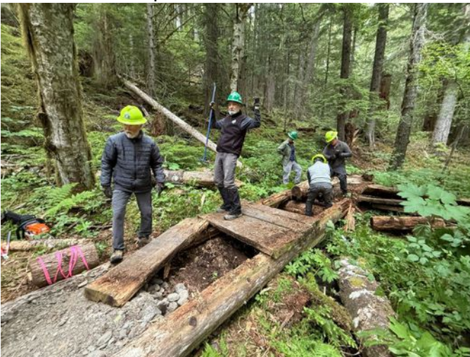
Demolition and spike removal
