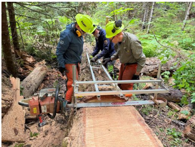
cutting decking with Alaskan saw mill
