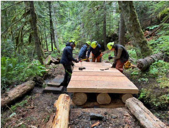
installing decking
