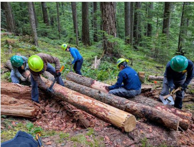
Debarking and moving the new stringers
