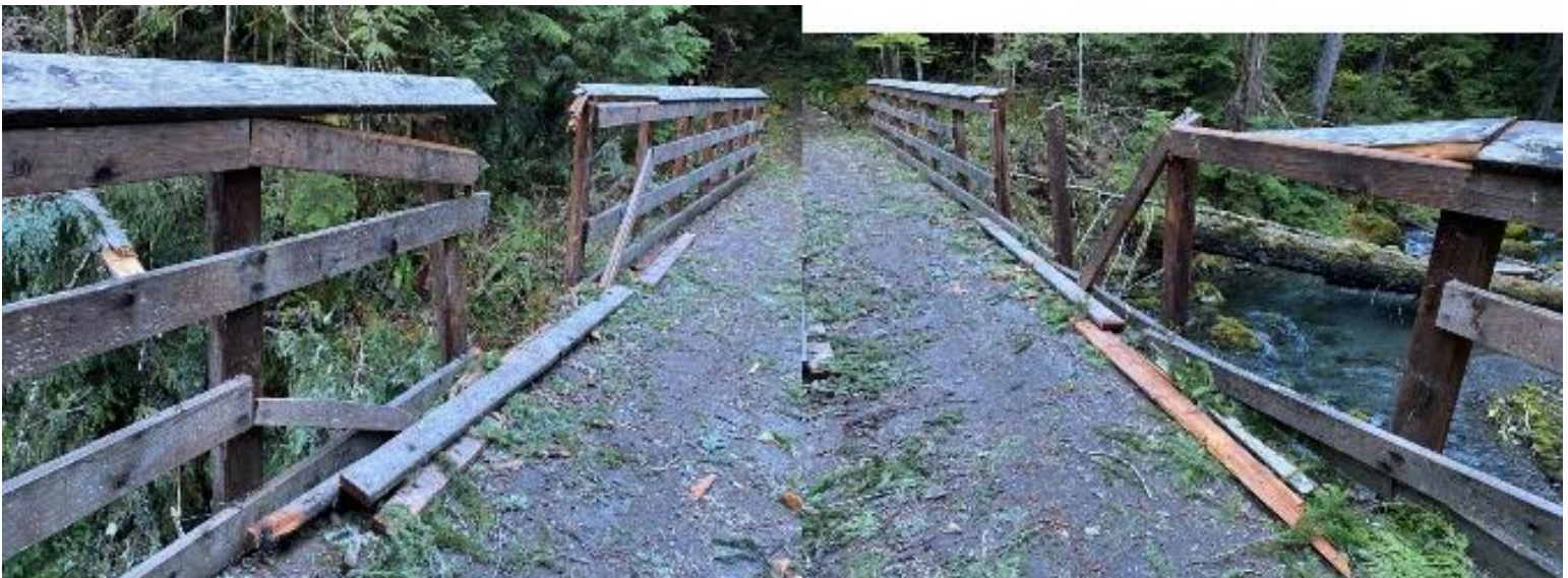
Railings were discovered in December to have been broken by a tree that fell on the bridge.
