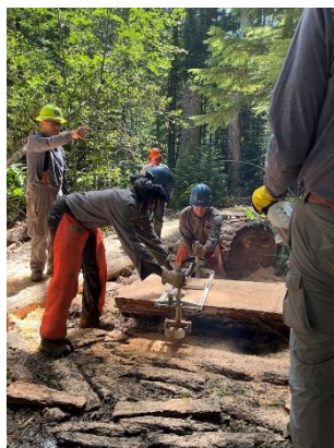
The youth crew got to learn how to use the Alaskan Saw Mill to make puncheon decking (for a different project)! Members of the Gray Wolf Crew were happy to help and teach them.
