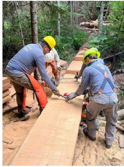
We cut along the log to where we left off with the debarking, with some following behind to tap in wedges. That keeps the long heavy cut plank from sagging and bogging down the saw. Then we cut off the plank at 5 feet, the width we need for the decking. Running the mill is a multi-person job.
