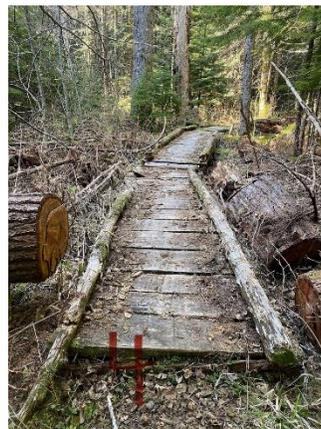
Left: the first puncheon that will be replaced by WTA. We cut 3 stringers, 2 bull rails and 2 sills for this. In addition – the big job – we made decking for it using the Alaskan saw mill.
