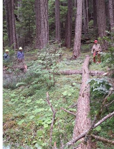
Lots of hunting around in the forest, cutting, and moving of logs to use for stringers, sills, bull rails and curb logs. Every one that we cut we also put a flag around it and marked on the end of it identifying what it is.
