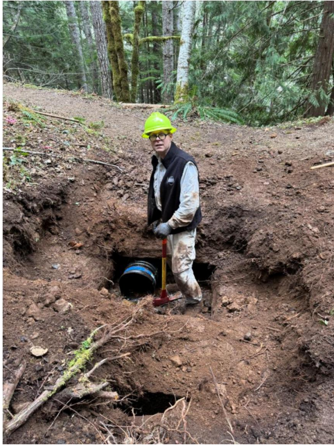
Culvert middle opened and pipe inserted
