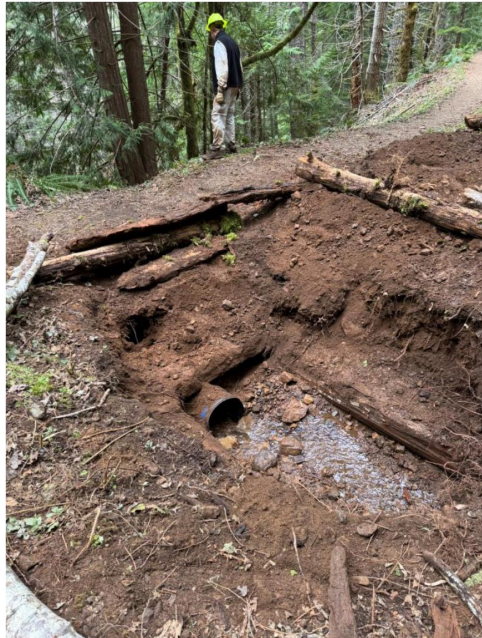
Culvert at close of work party
