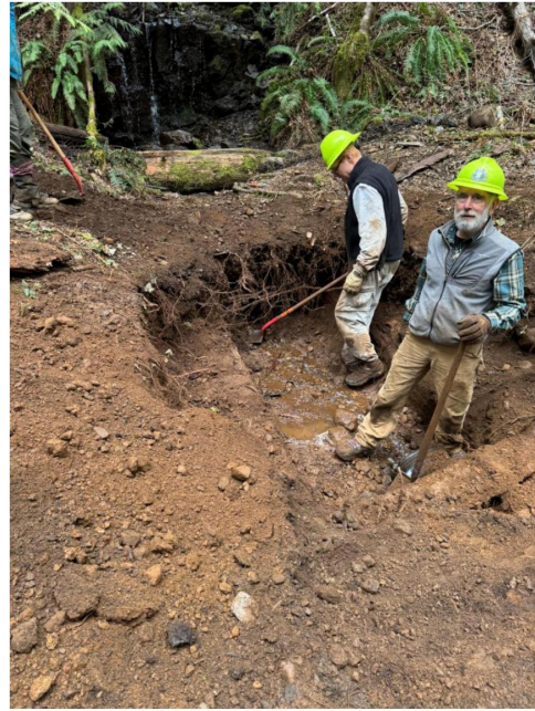
Further opening culvert
