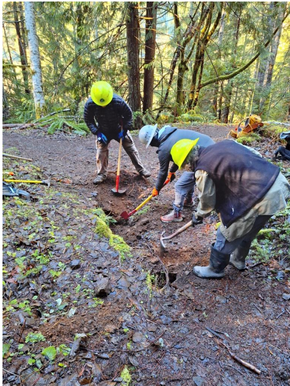
Working to open sinkholes
