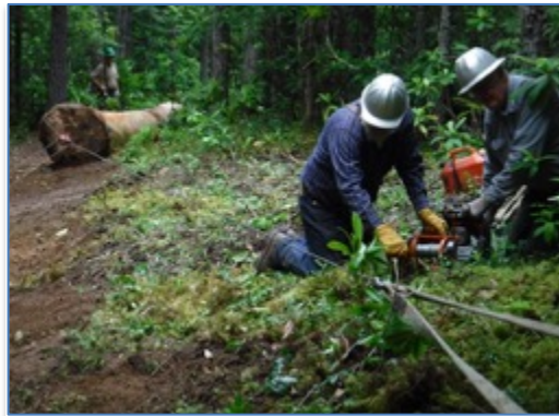
Moving log with rigging.
