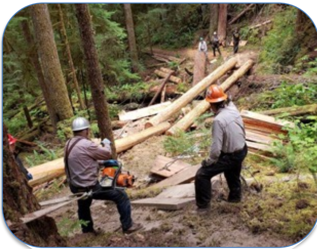
Moving stringer into place with chain saw winch, Aug. 2019
