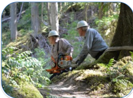
Moving stringer into place with chain saw winch, Aug. 2019
